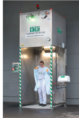
Tanknotduschen Tank safety showers
